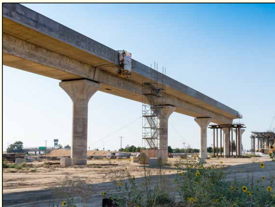
The 3,700-foot Cedar Viaduct will carry high-speed trains over State Route 99, North Avenue, Cedar Avenue, and Golden State Boulevard.
